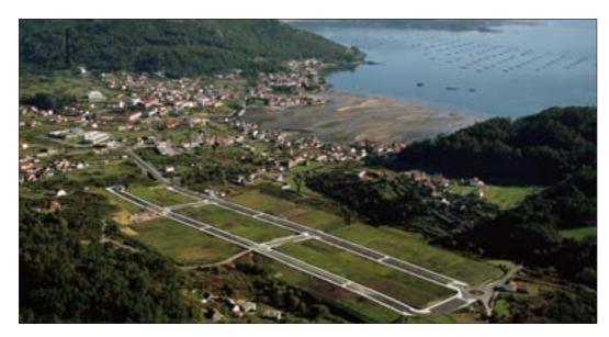
Two longitudinal and two transversal roads, with a 23 meter-section were built, plus two 3.5 meter-wide lanes, parking facilities and two 3 meter-wide sidewalks. A traffic circle, 800 meters-long and 11 meters wide, from the AC-400 road provides access to the business park.
