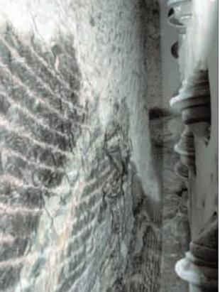
THE DOUBLE-SHIELD MIXED TUNNELLING machine that was used has a 9.5 m excavation diameter on the west side, and 9.46 on the east side. In the photograph, the front of the tunnel and detail of the head of the tunnelling machine.
