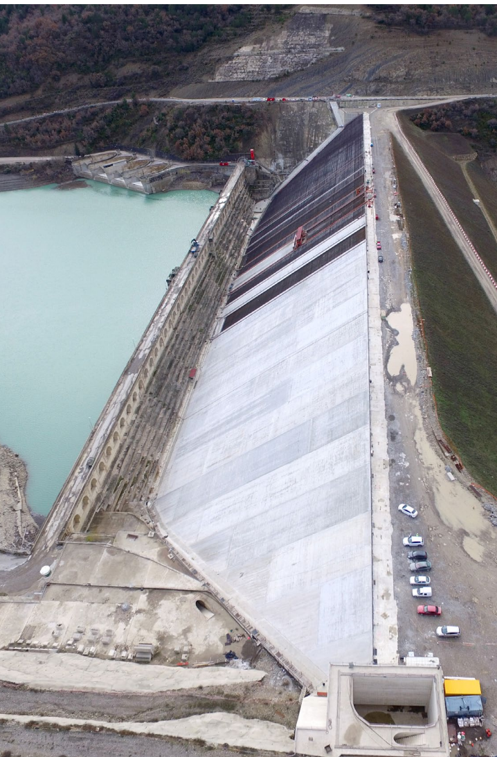
Yesa dam, Navarre (Spain).
