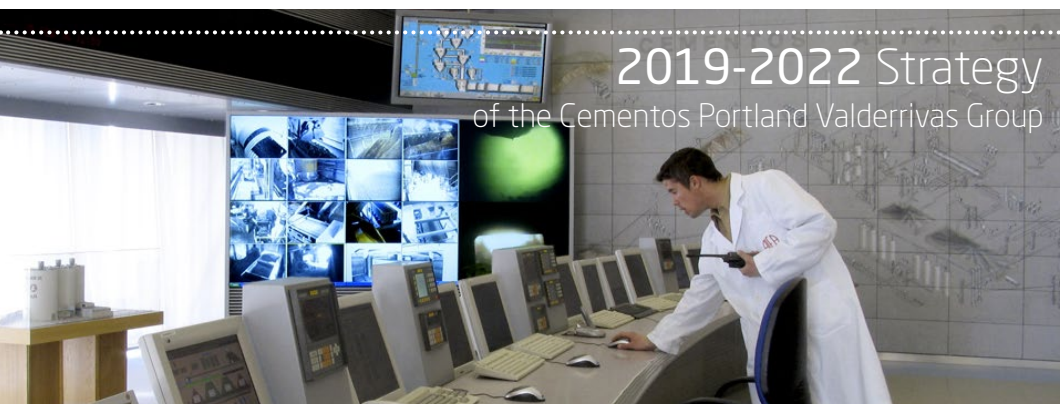
Control Room at the Mataporquera factory in Santander (Spain).
