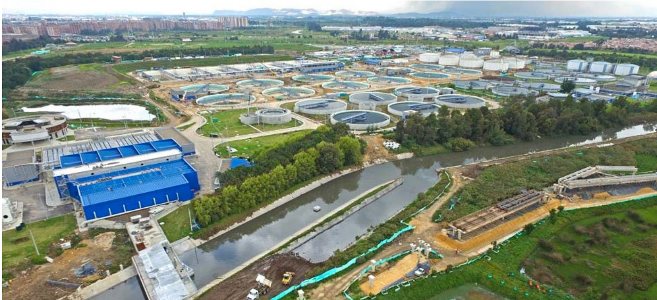
"El Salitre" wastewater treatment plant (WWTP) in Colombia.
