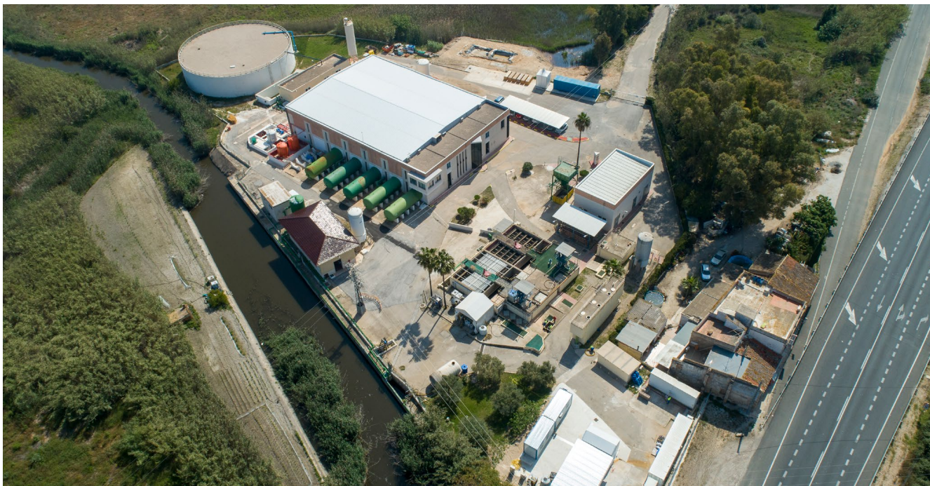
The MIDES project, led by Aqualia, operates the first two desalination plants that are wholly energy self-sufficient in the world, in Dénia (Alicante, Spain) and Guía de Isora (Santa Cruz de Tenerife, Spain).
