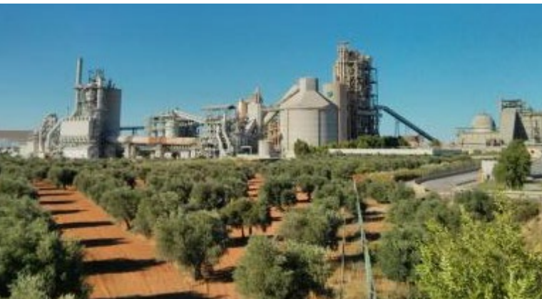
Panoramic view of the El Alto factory, Madrid (Spain).
