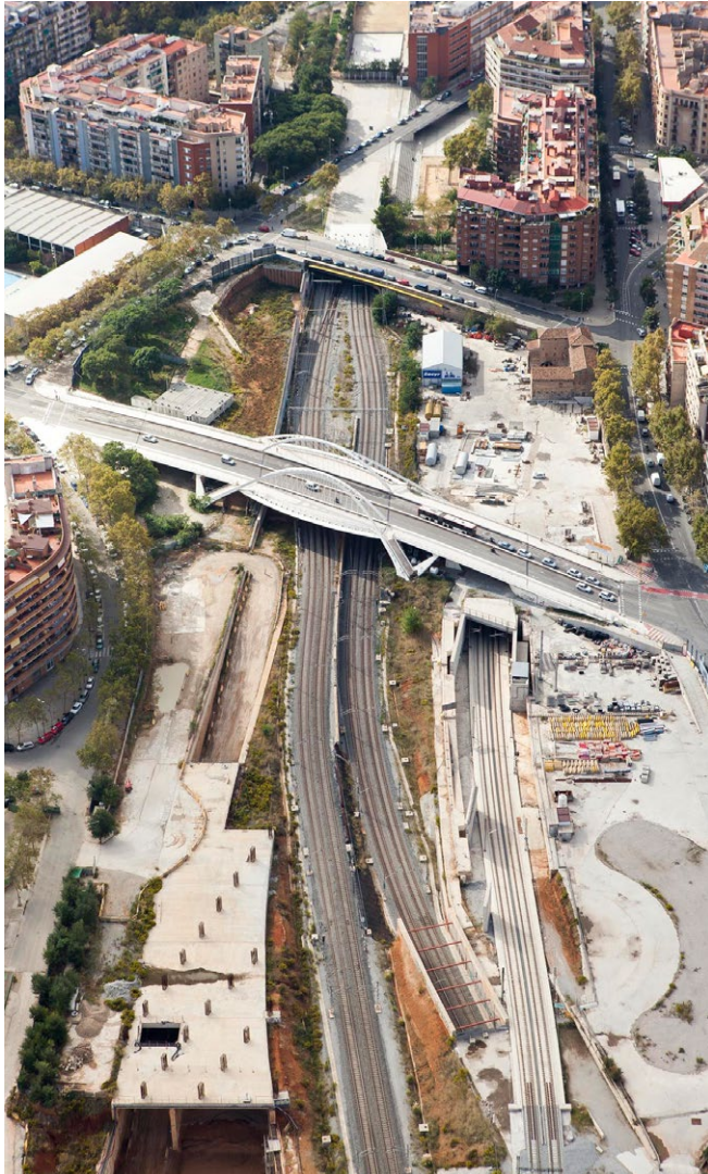
Accesses to the Sagrera station
