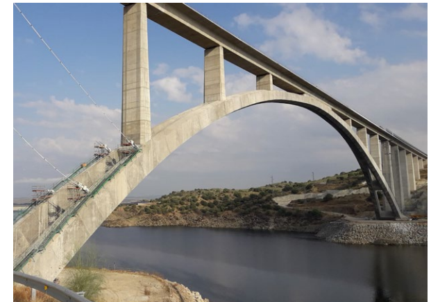
Almonte Viaduct, Caceres (Spain).
