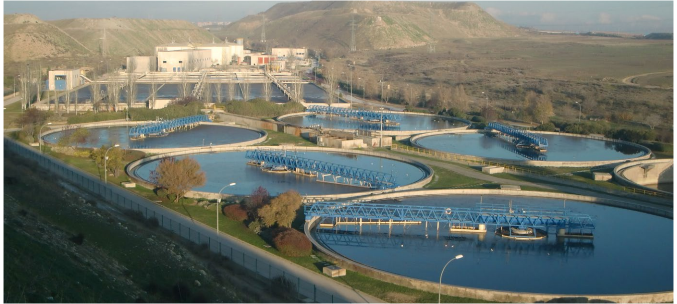
EDAR (Waste Water Treatment Plant) of La Gavia, Madrid, Spain
