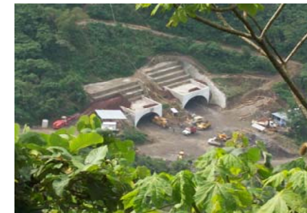
Xicoteppec Tunnel in Mexico
