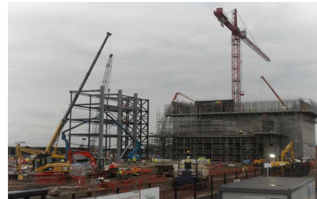
Building in progress (Feb. 2012)
