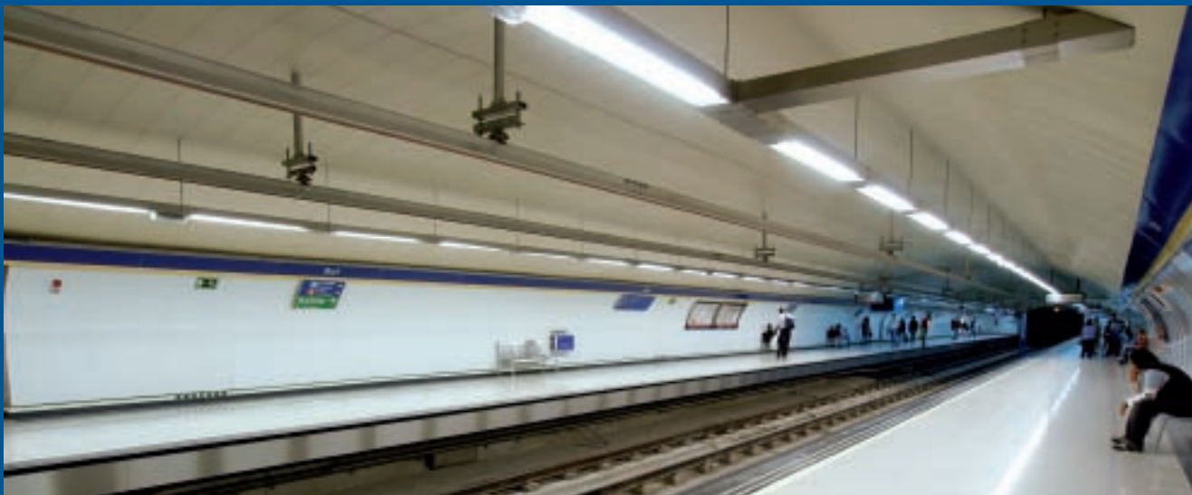
Larger platforms at underground line 3's Sol station. Madrid
