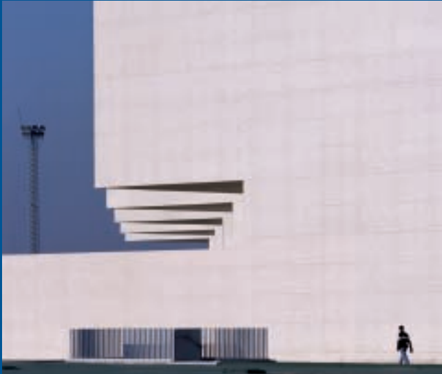
Delicias intermodal transfer facility, Zaragoza. 2006 Award to Foster Quality
