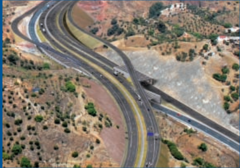
Málaga west ring road. Section connecting road C-3310 to the A-7 Autovía del Mediterráneo dual carriageway. Málaga
