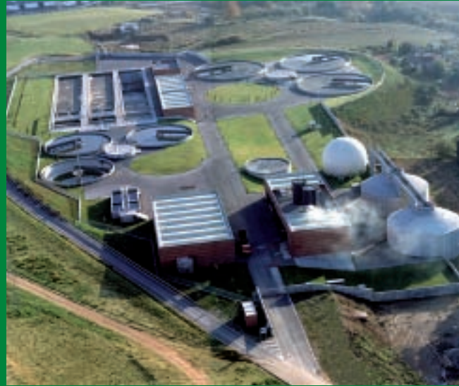
Sabadell purifying plant (SPA). Barcelona
