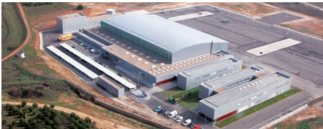
Civil Guard helicopter air base. Torrejón de Ardoz. Madrid
