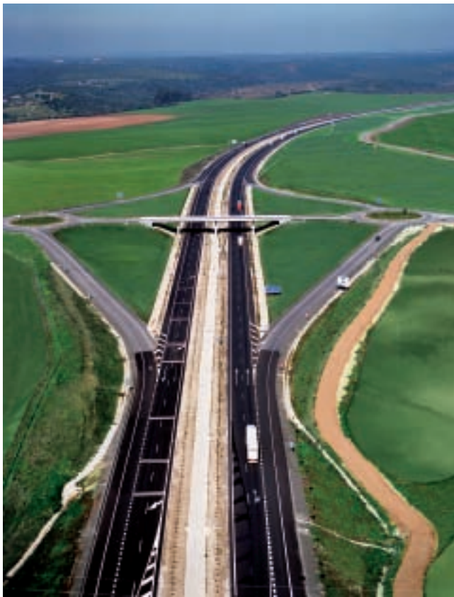
Autovía de La Plata dual carriageway. Gerena-Camas section. Sevilla
