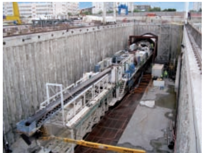
Extension of Madrid underground line 7. Coslada-San Fernando section
