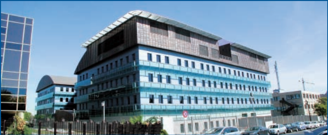
Offices of the Directorate-General of Traffic, Madrid
