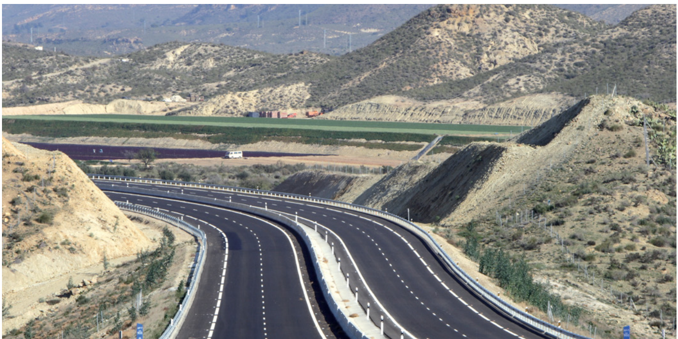
Canero Viaduct. Cantábrico motorway, Querusas - Otur section
