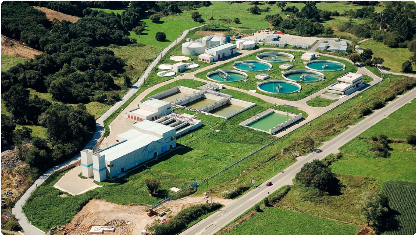
WASTEWATER TREATMENT PLANT, SAN PANTALEÓN, SANTANDER.
