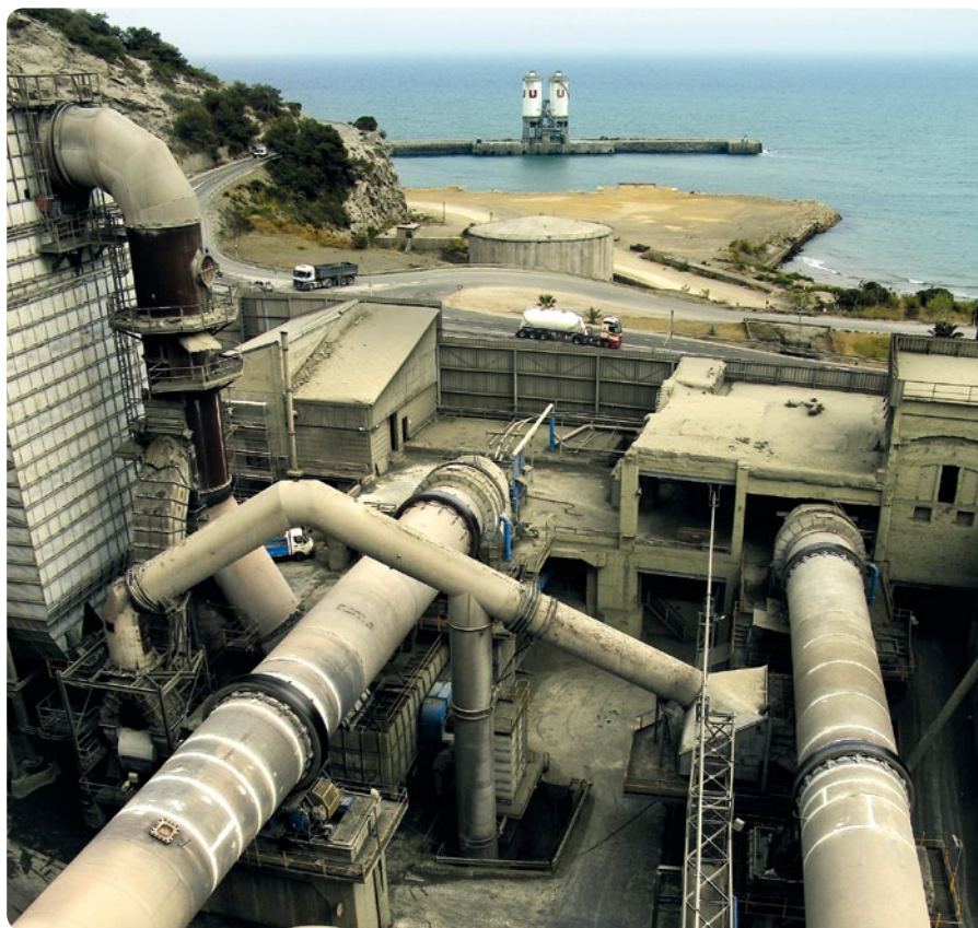
CEMENT FACTORY IN VALLCARCA, BARCELONA.
