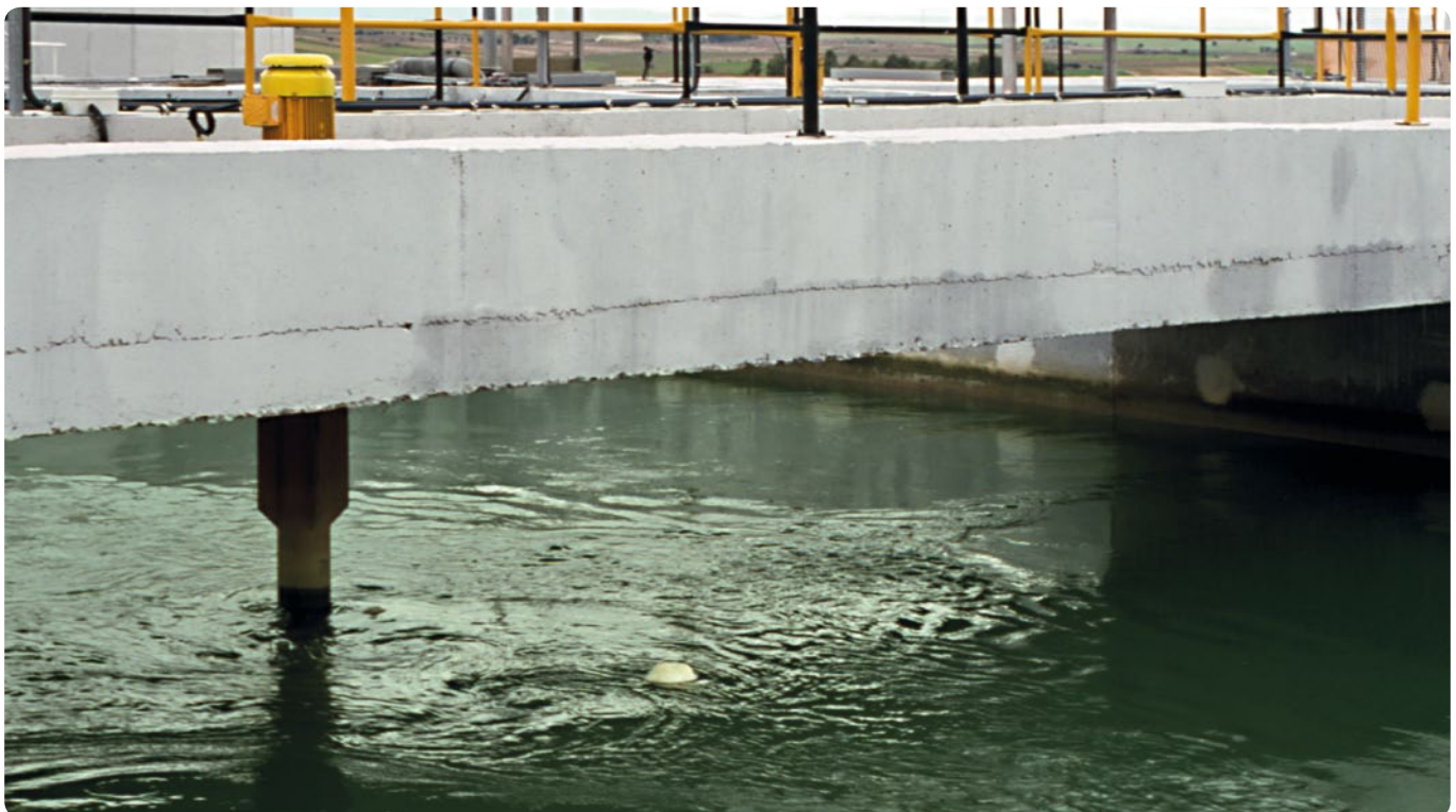
DRINKING-WATER TREATMENT PLANT, VALMOJADO, TOLEDO.
