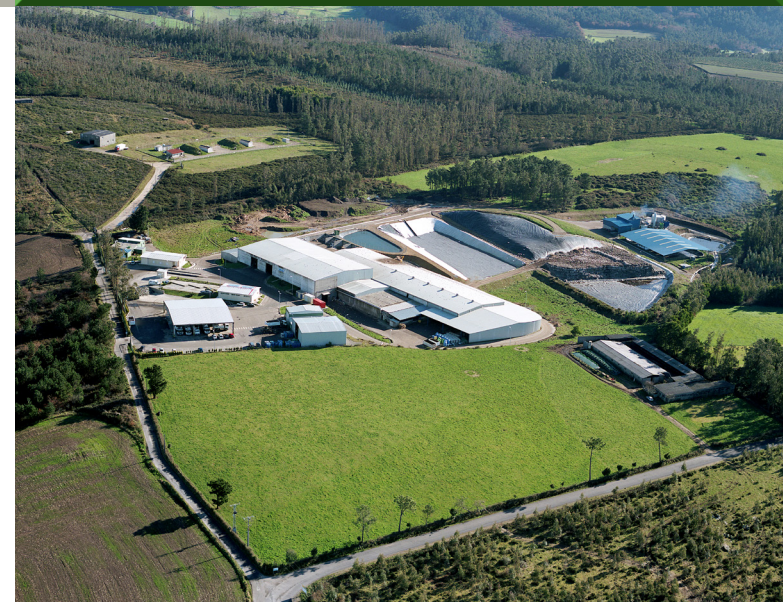
Center for solid waste treatment, Barbanza, La Coruña.
