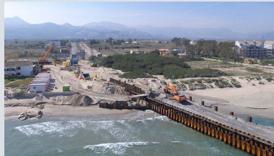
Denia Landfall 3. Underwater gas pipeline
