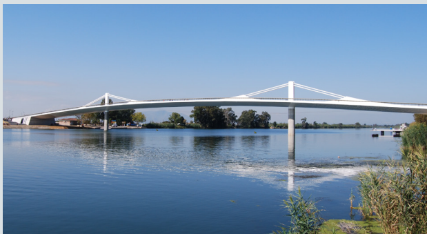
Ebro River Bridge, Deltebre
