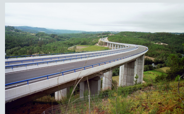
Viaduct over the Ulla River, Galician Motorway
