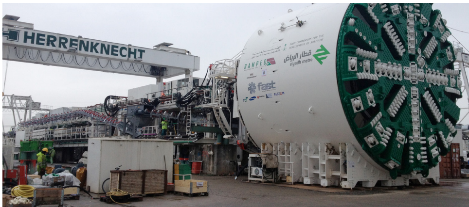
Tunnel boring of Riyadh Metro (Saudi Arabia).
