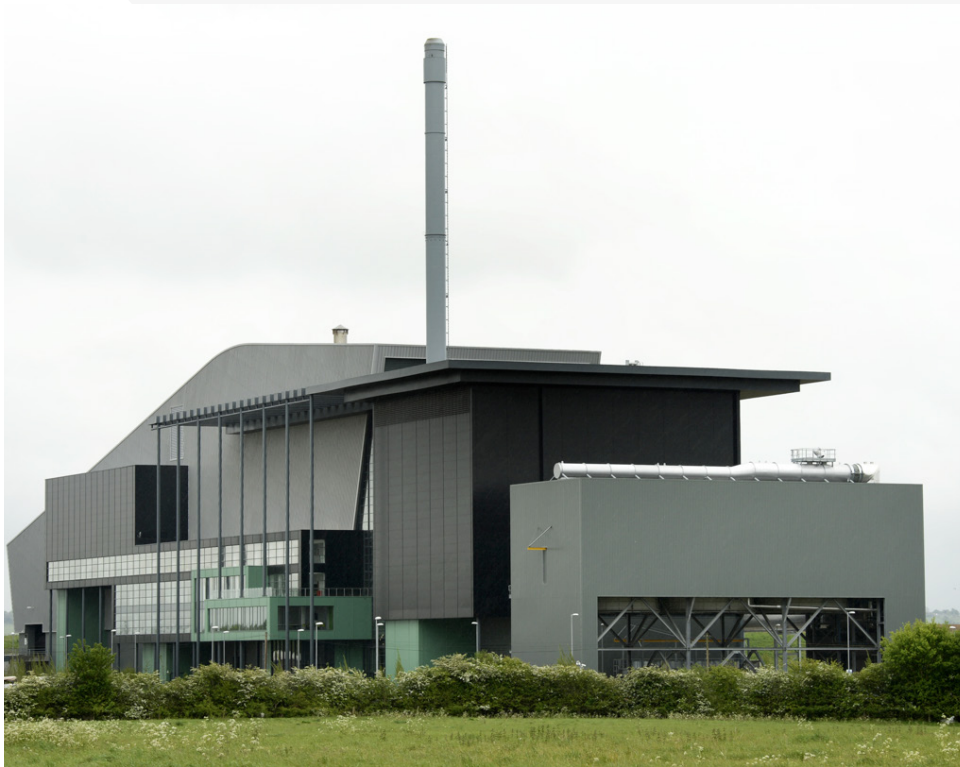
Incineration plant in Lincolnshire (United Kingdom).
