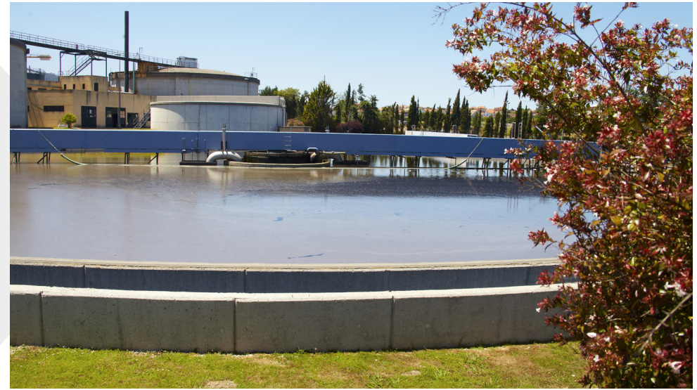
Vigo Wastewater Treatment Plant (Spain).
