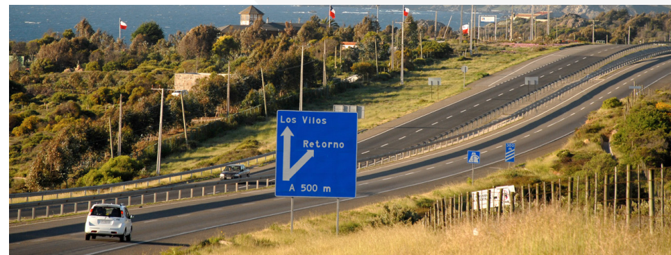
Aconcagua Motorway (Chile).
