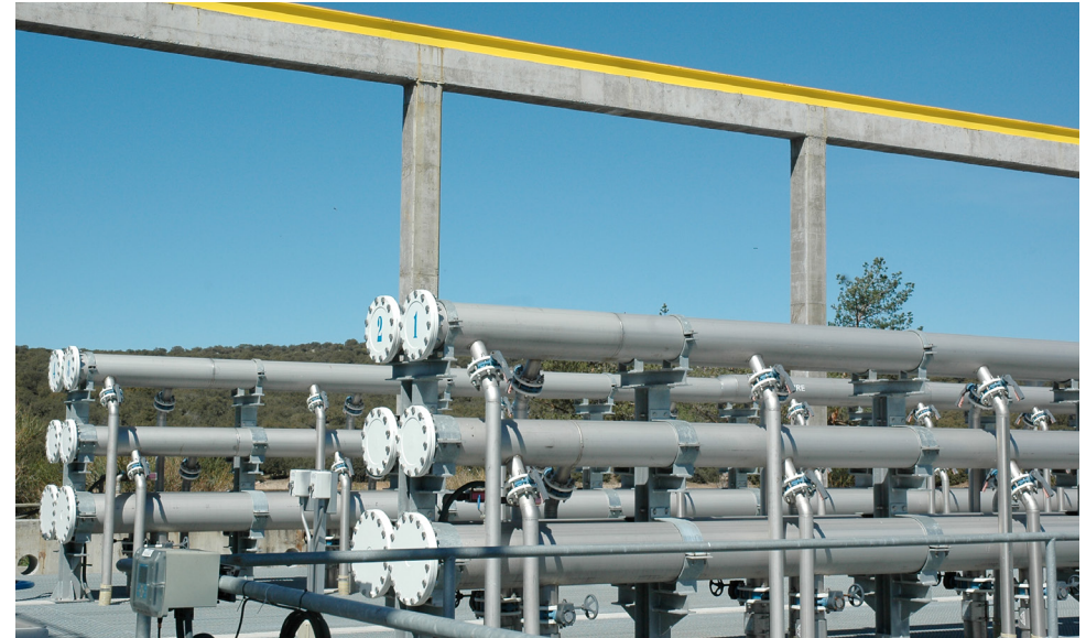
Ultrafiltration membrane bioreactor (MBR).
