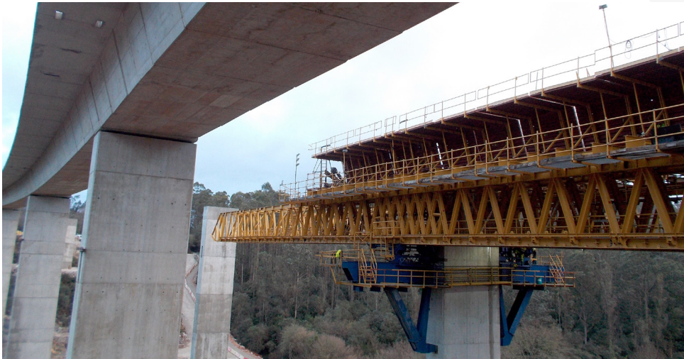
Viaduct over the River Cabra. Cantabrian Highway (Spain).
