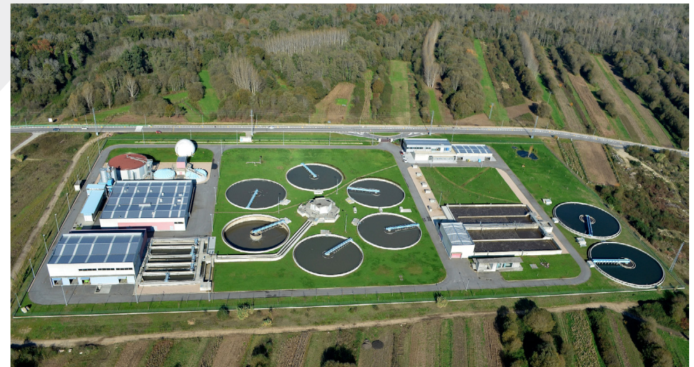
Guillarei Wastewater Treatment Plant in Tui (Spain).
