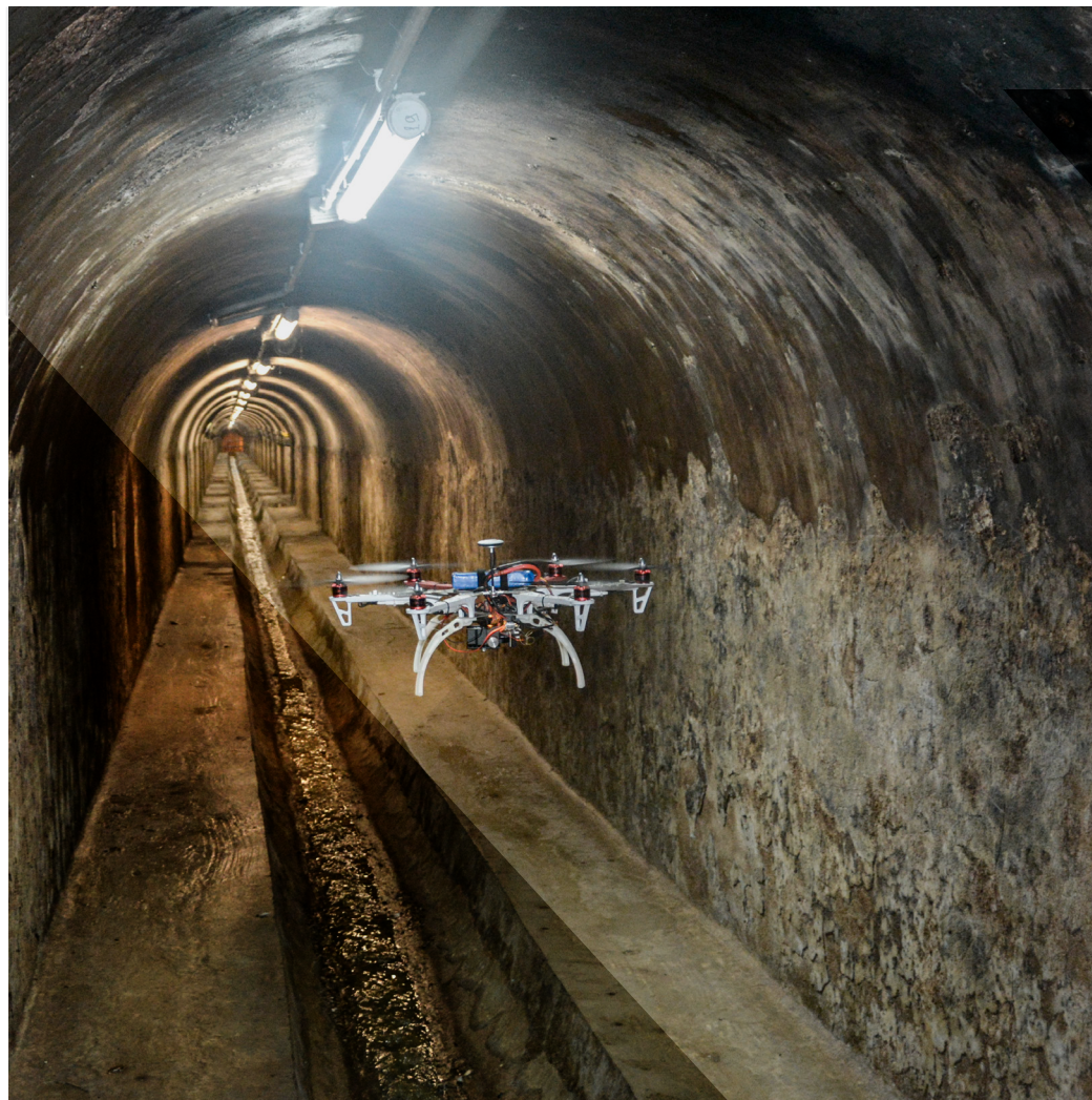
A drone examines the sewage system of Barcelona (Spain).
