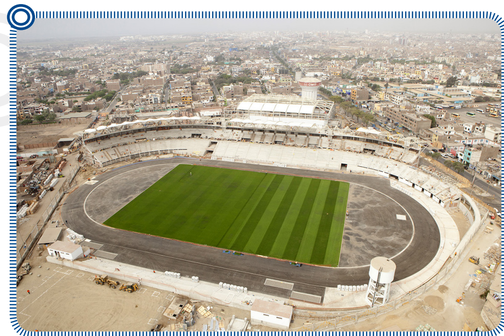
Sports complex in Trujillo (Peru)
