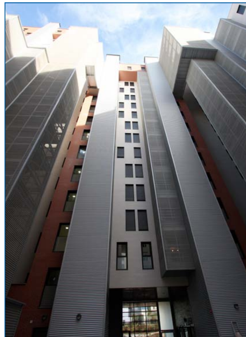
Homes in Móstoles (Madrid)
