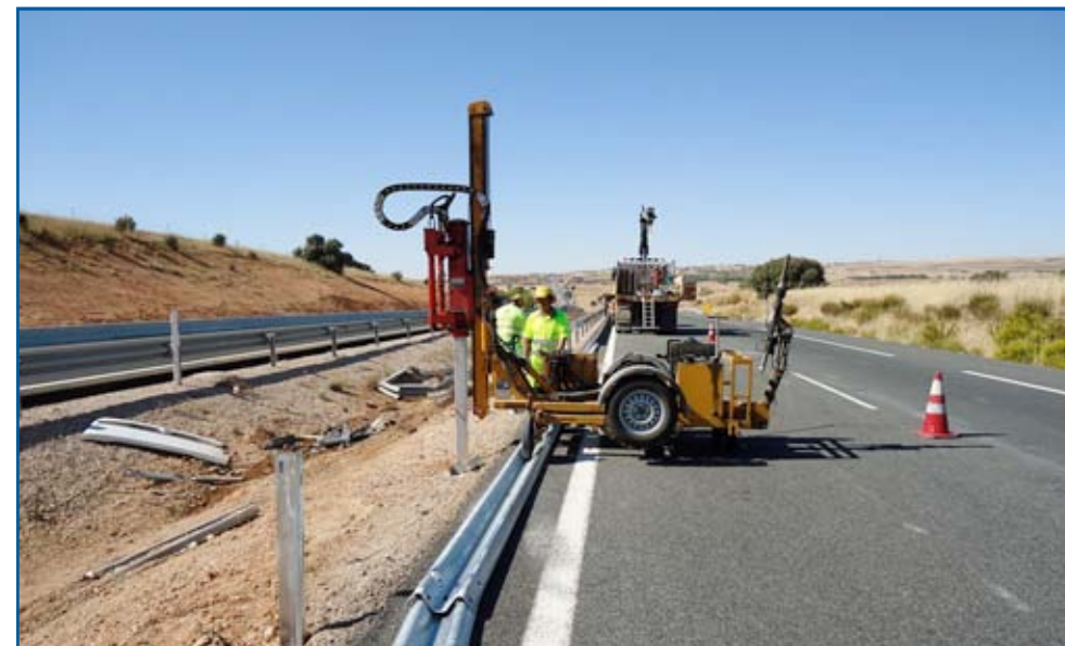
Installing safety fences on highways
