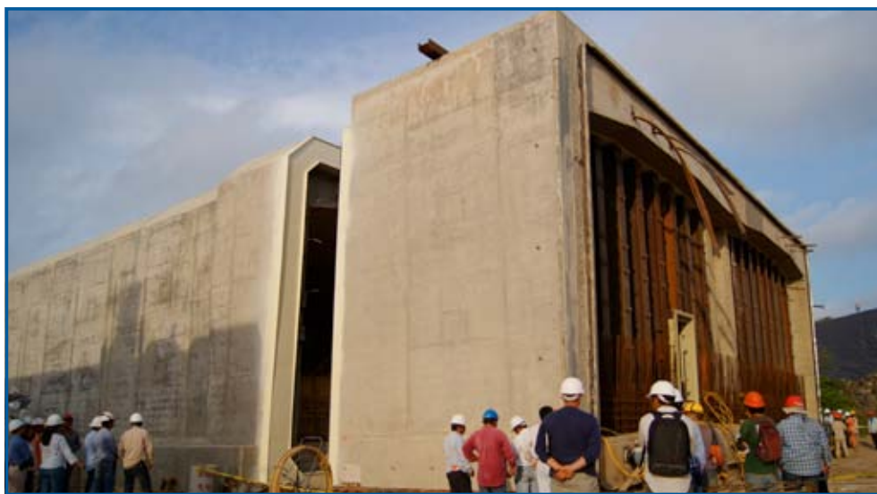
Coatzacoalcos Tunnel, Mexico
