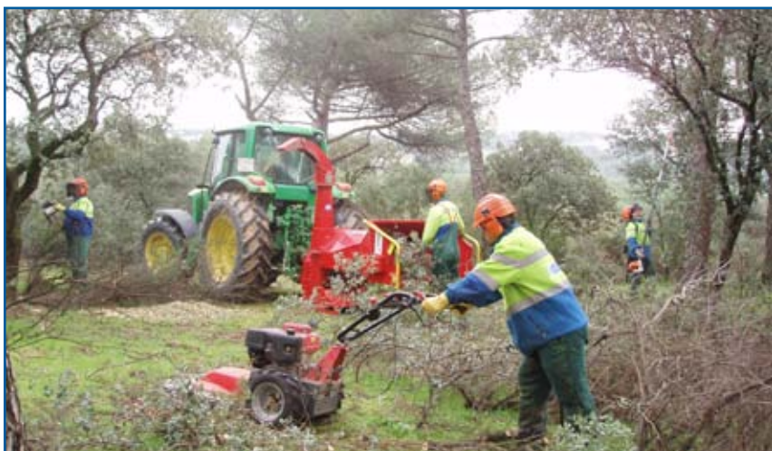
Crushing and clearing works
