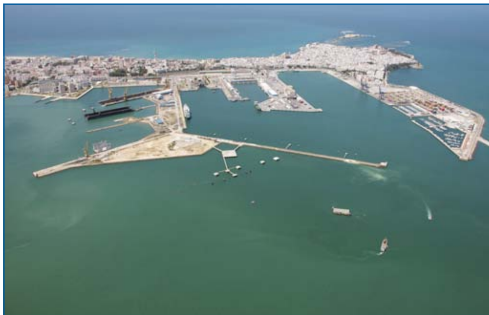
Cadiz Port Container Terminal
