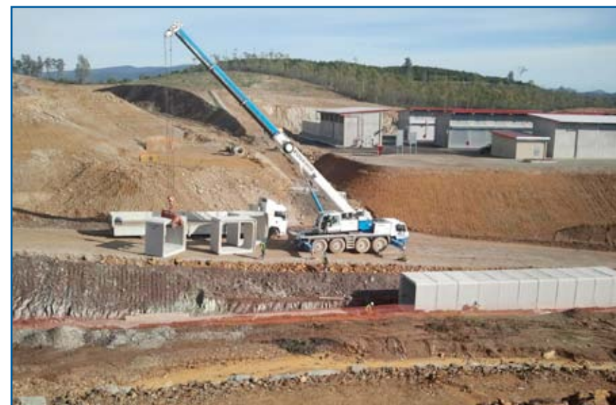
Placement of modular reinforced concrete structures
