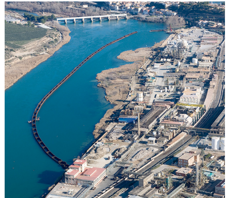
Decontamination of Flix Reservoir, Tarragona
