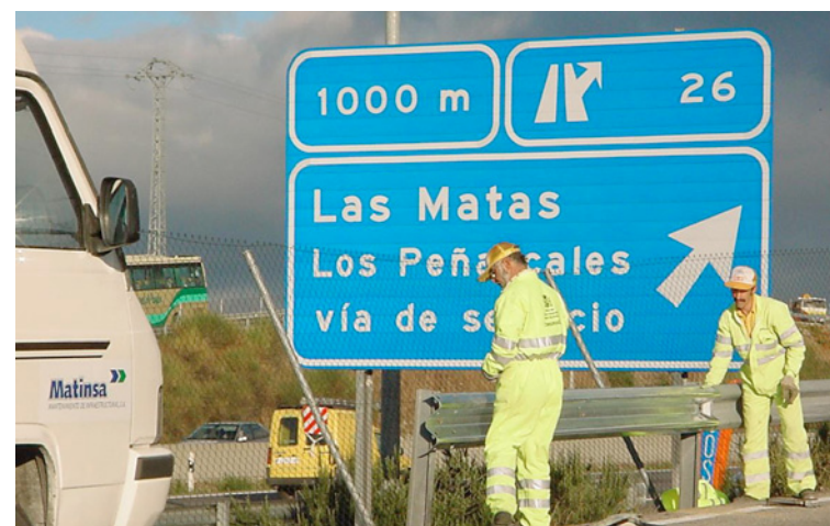
Installing a metal barrier
