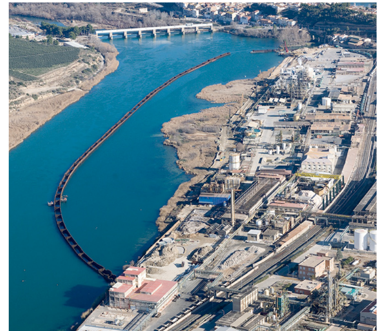
Decontamination of Flix Reservoir, Tarragona
