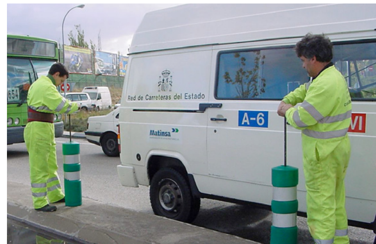
Installing a flexible bollard
