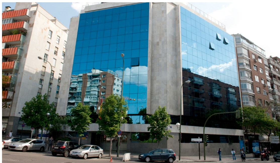
Road Infrastructure's General Direction headquarters rehabilitation, Madrid
