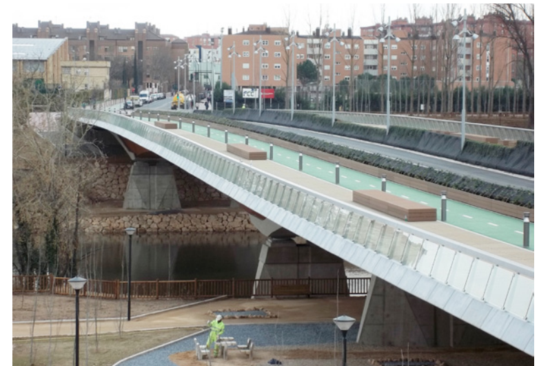
Bridge over the Pisuergra River, Valladolid
