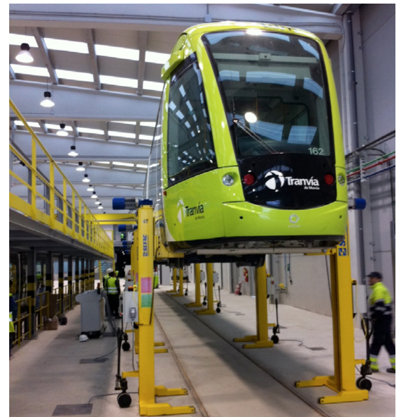
Tram maintenance facility
