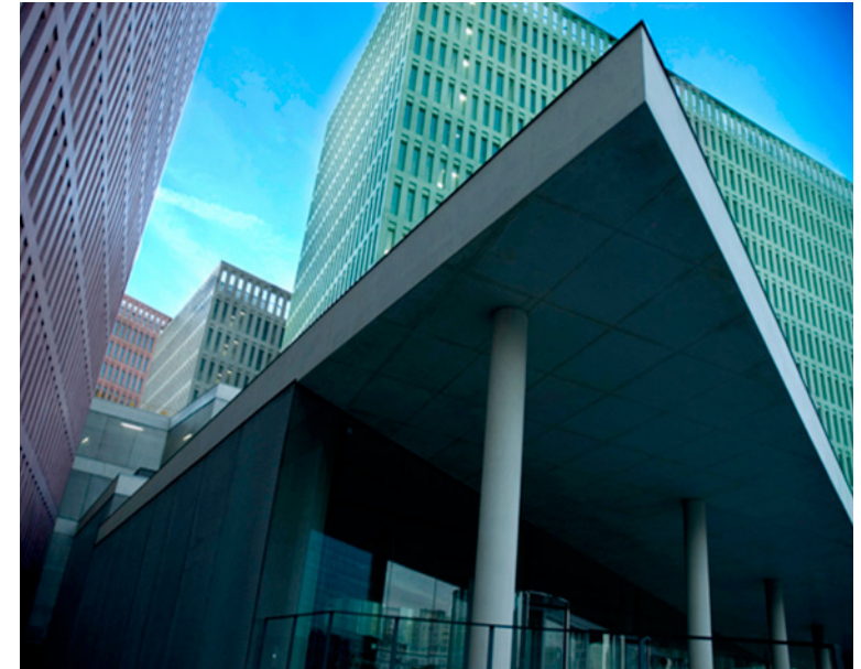
City of Justice complex in Barcelona
