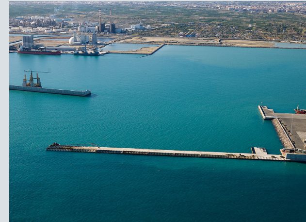
East Dock, Castellón Harbour
