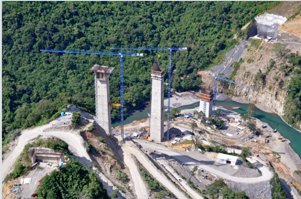
Piers for San Marco Viaduct, Mexico
