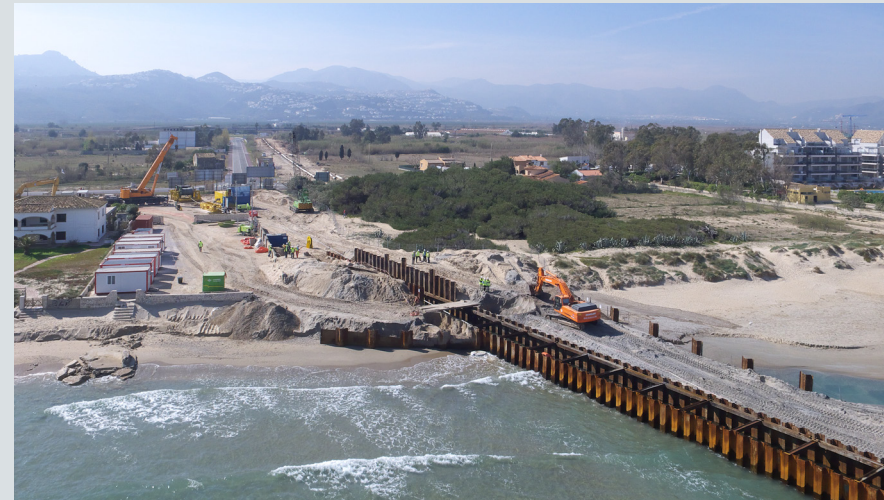
Denia Landfall 3. Underwater gas pipeline
