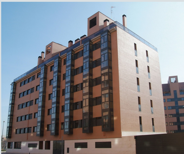
Housing in the northern area, Las Tablas, Madrid
