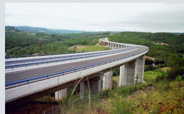
Viaduct over the Ulla River, Galician Motorway
