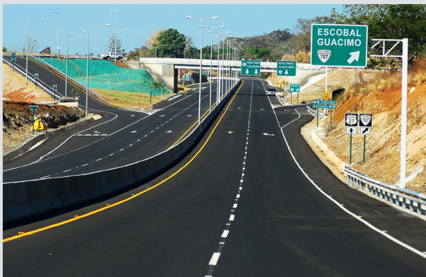
San José Caldera Motorway, Costa Rica
