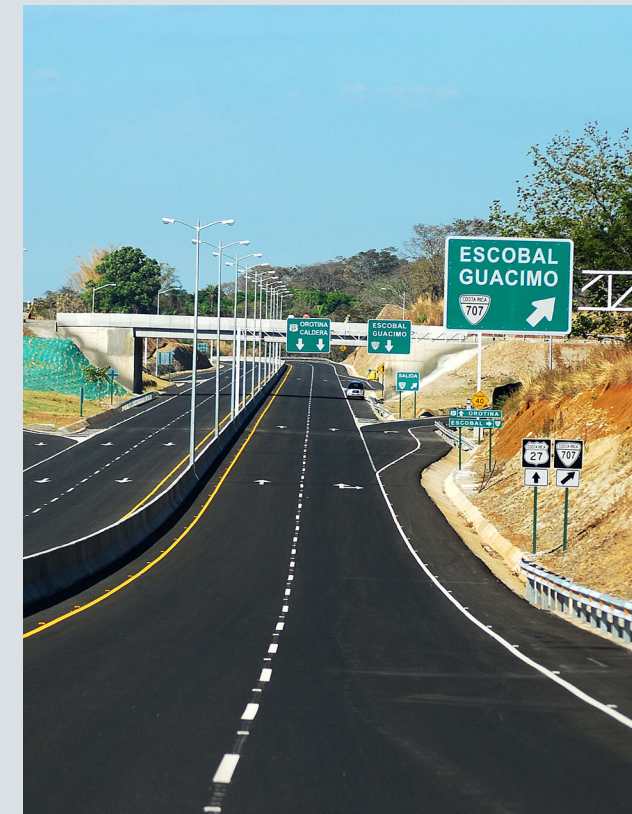
San José Caldera Motorway, Costa Rica
