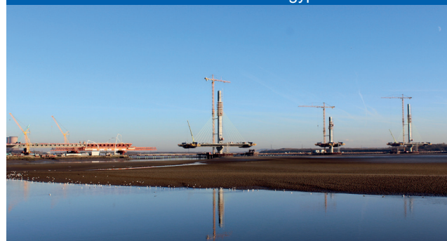
Bridge of Mersey. United Kingdom.
