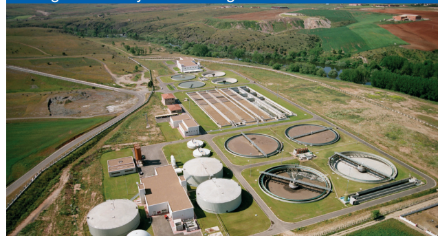
Wastewater treatment plant in Salamanca. Spain.
