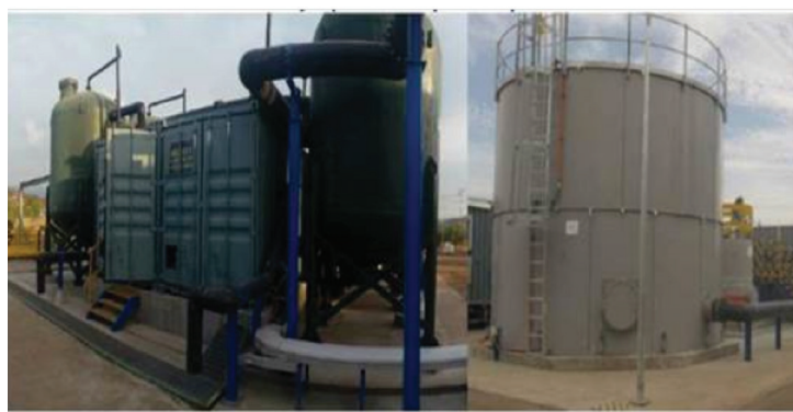
Sand filters and runoff tank.
